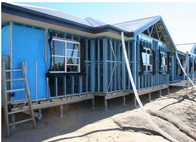
The Narrabri Abbeyfield house under construction.
